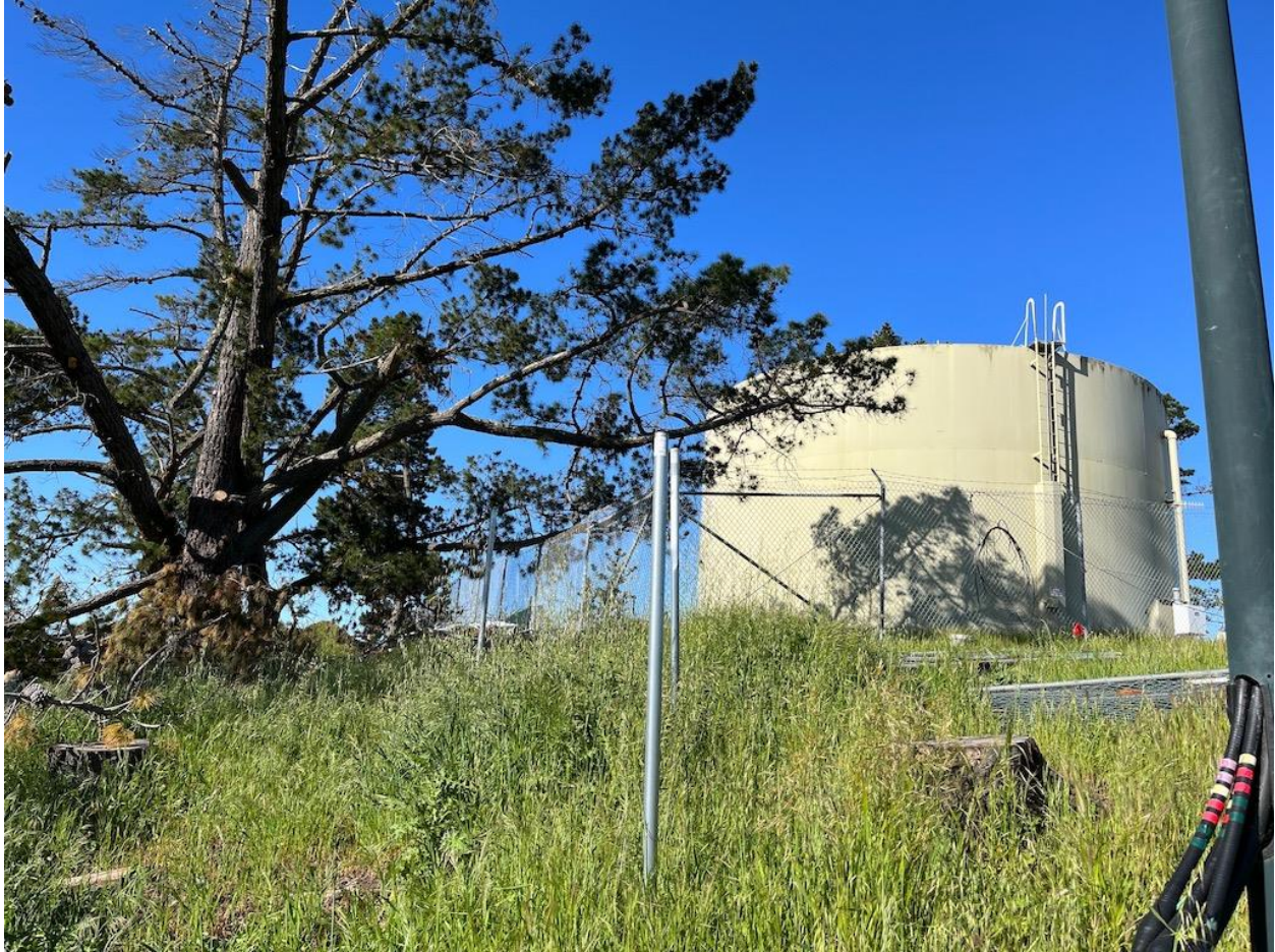
Figure 6. Existing Trees and Fencing, looking South.
