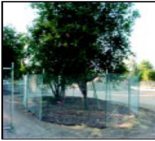
IMAGE 2.15-1 Tree Protection Fence at the Dripline
