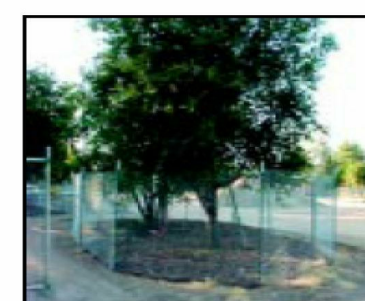
IMAGE 2.15-1 Tree Protection Fence at the Dripline
