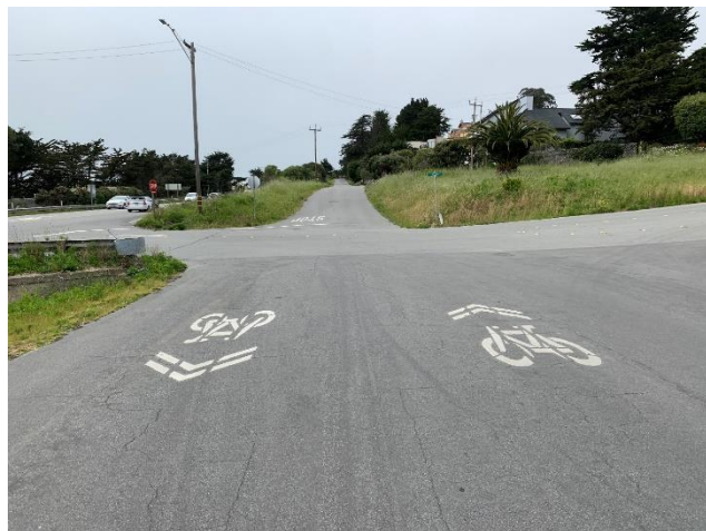
Class III Bike Route with Sharrows on Carlos Street in Moss Beach
